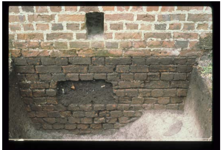
Figure 61: Views of opening in north foundation as excavated by Lewis in 1980 (right); Expanded excavation in 2007 and associated Feature 4.
