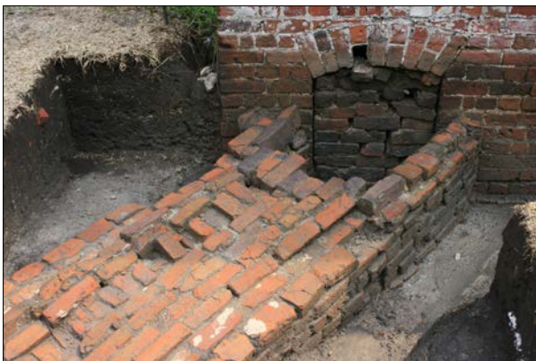
Figure 56: Views of interface of vault opening and drain. The opening was bricked after the 1980 excavations to stabilize the building and soils inside
