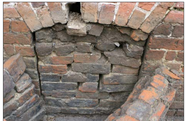
Figure 56: Views of interface of vault opening and drain. The opening was bricked after the 1980 excavations to stabilize the building and soils inside
