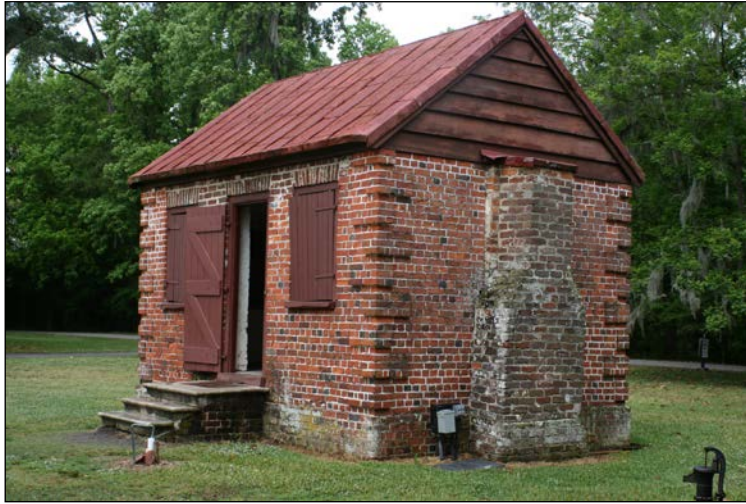
Figure 2: the privy before excavation. View shows the east side of the building. The 19 th century chimney stack is visible. Note also the electrical boxes and water lines along the eastern side of the structure.
